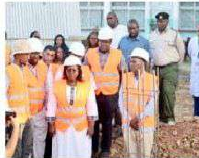
CS Peninah Malonza (Second Right) accompanied by PS Kello Harsama (Right) inspects the construction of the ICU facility at the Malindi Sub-County Hospital.
